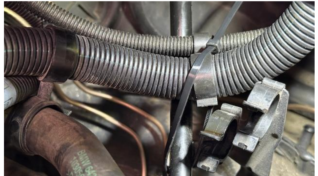
40. Use a cable tie to secure the dipstick around the conduit cable as shown.
