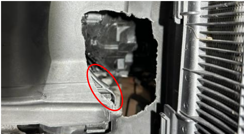
7. Using a dremmel or similar, cut around the marked line and use the rubberised edge as a guide to cut the complete opening. Be careful of the mount behind the panel as circled.
